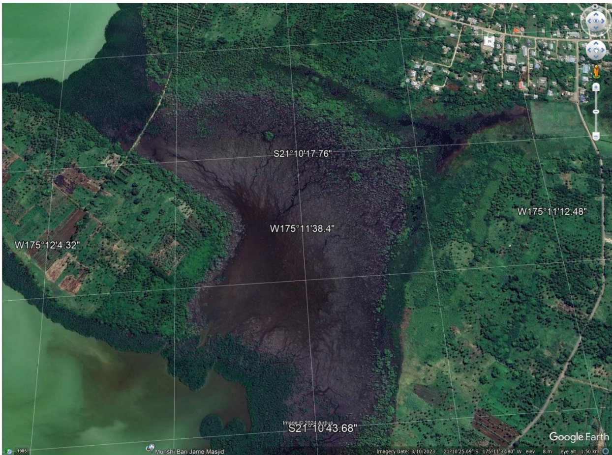
Nukuhetulu mangrove forest, Tongatapu in 2023 (Google Earth Pro 2024), showing die-off of 100 hectares attributed to road construction, interrupted tidal flow and poor water flushing (Tonga Geological Services 2023)
