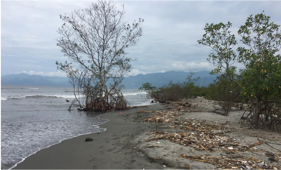
Mangrove cover loss and substrate erosion due to rising sea level and earthquake in the Cuyamel community, Honduras, near the Guatemala border (photo credit: Lenin Corrales).
