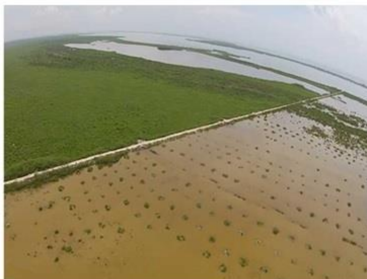
Panoramic view of road construction effects in El Playón with visible restoration efforts (green points). (photo credits: OIN, 2015).
