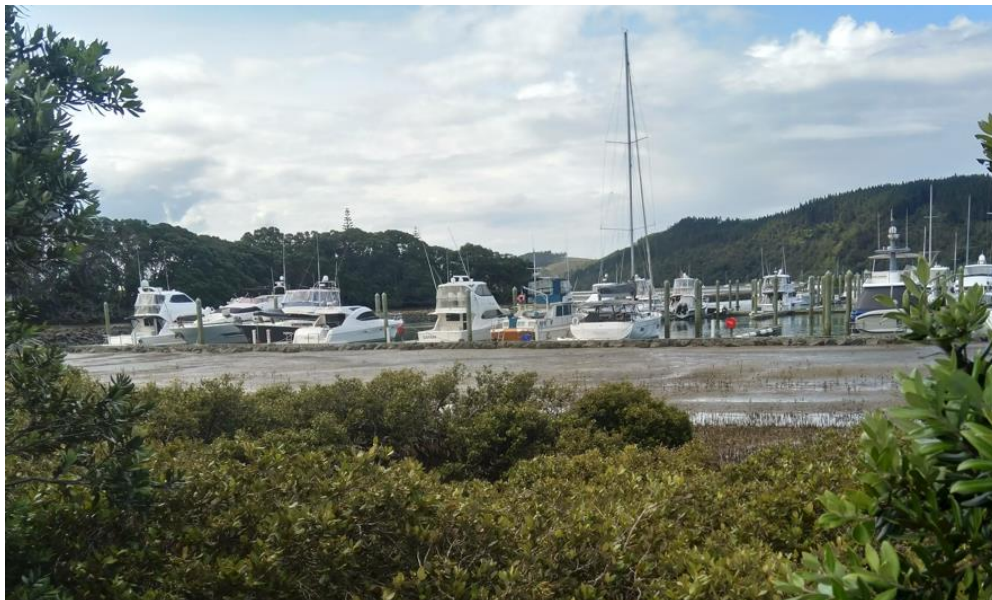
Mangroves invading mudflats created following the construction of a marina, Whangamata, Coromandel Peninsula (Photo credit: Jeffrey McNeill)
