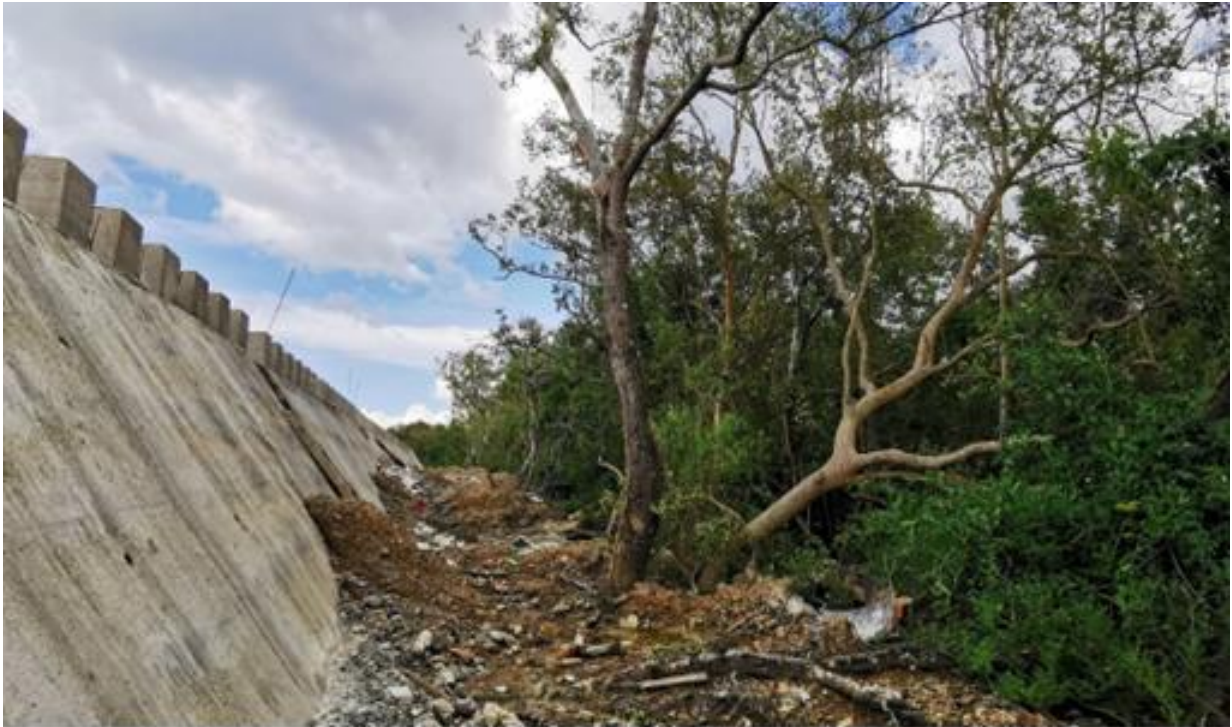
Mangrove forest destroyed during coastal road construction in Marinduque Province, Philippines (Photo credit: Dixon Gevaña).
