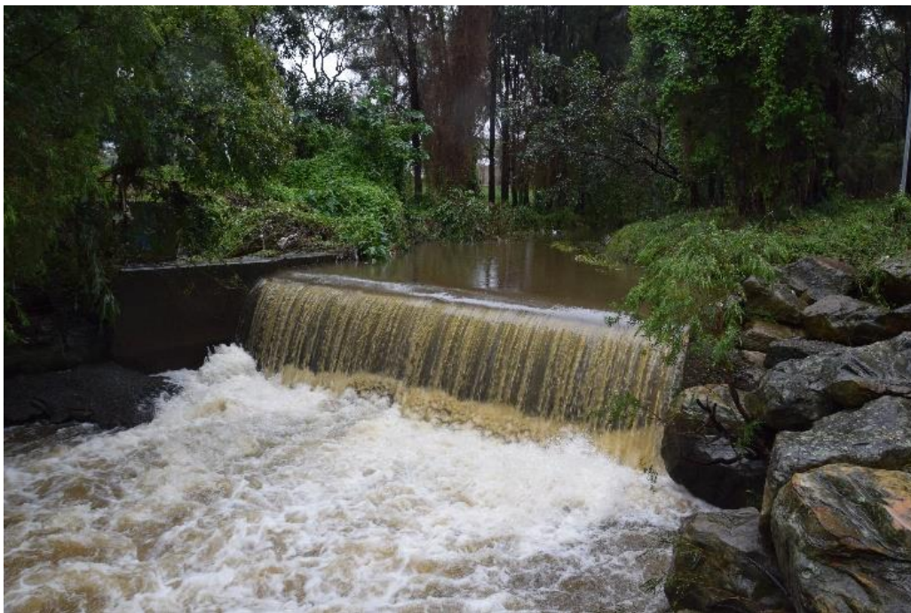
Above: the weir/creek crossing under normal flow conditions.
