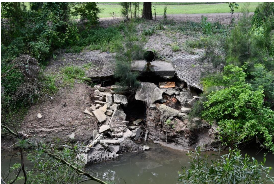
Above: geotextile mattress on the eastern creek bank, photo taken in December 2021.
