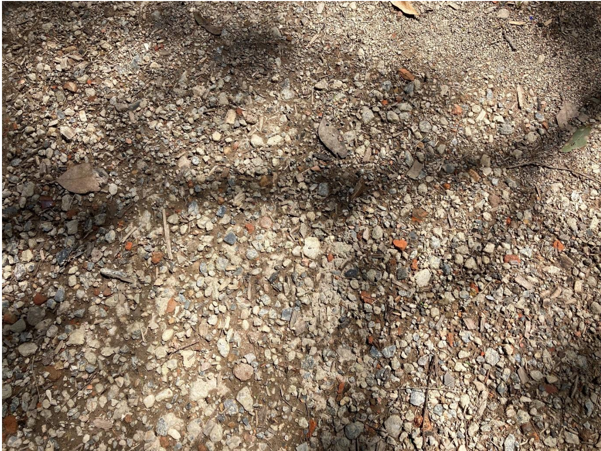
Close up of the central split path in mid-October 2022, showing the hardened, heavily compacted layer of mulch, gravel and clay.
