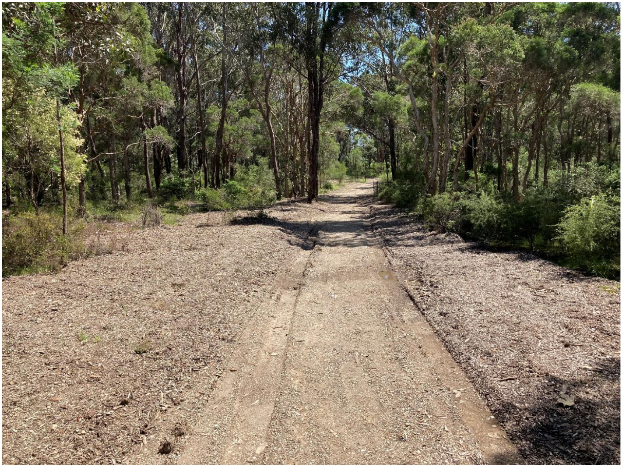
Above: the central split path in late September 2021, pre-works.
