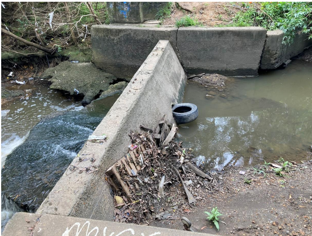
Large quantities of debris and rubbish, including a tyre, shopping trolley, wooden pallet, and various plastic items, altering the water flow at the creek crossing and polluting the water.
