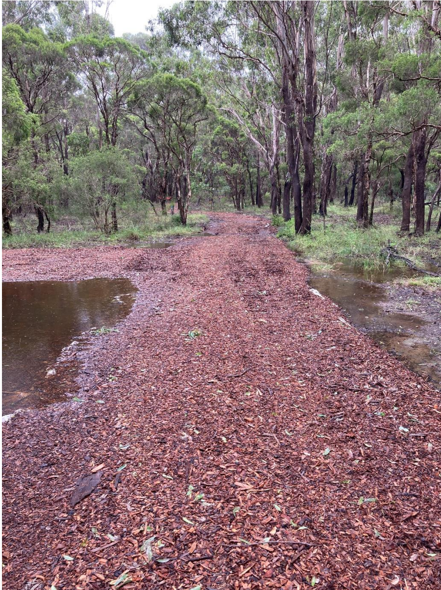
Initial laying down of mulch along paths in the reserve.
