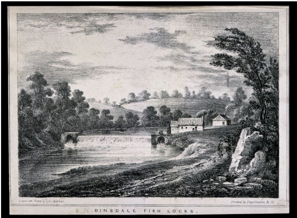
Figure S2. View of the weir and fish locks (each side of weir) on the River Tees at Dinsdale (18 km upstream of tidal limit) in the early 19th Century, drawn by J.M. Sparks.
