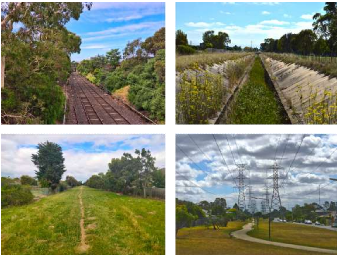
Figure 1. Example of the easement types included in the study, including (a) railway, (b) disused open sewer and (c) underground drainage pipeline, and (d) high-power transmission lines.
