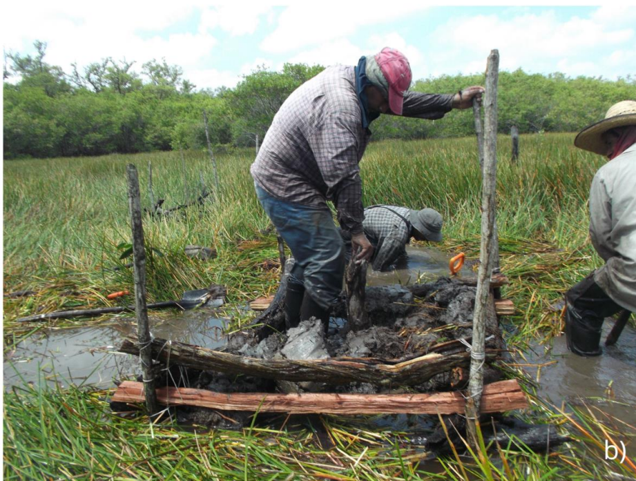
Figure 7a. a) Construction and securing of the chinampa structure; b) Filling the structure with adjacent sediments and compacting them.
