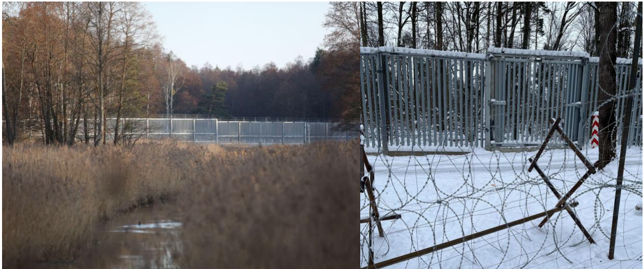
Fig. 2: Fenced Narewka River (left), one of seven transboundary rivers in Białowieża Forest, and one of the 24 gates (right) installed in Poland’s 186-km barrier to enable wildlife movement (of those, 9 such gates are in Białowieża Forest, which is bisected by the border for 53.4 km).
